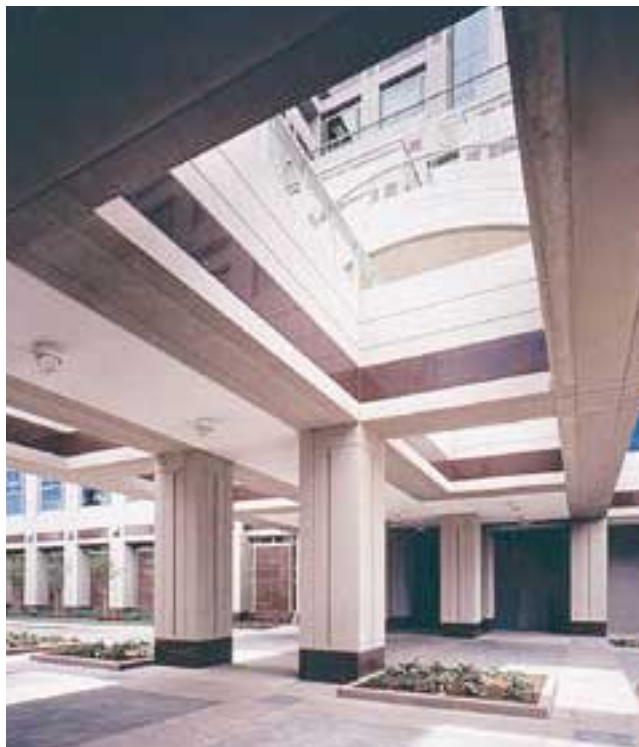
Fig. 9. A special panel cart was used to deliver precast panels to this area, where panels had to be set 36 ft (11 m) back under the second floor overhang.
