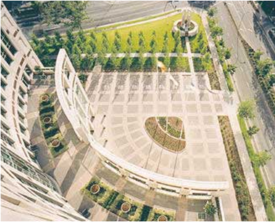
Fig. 11. Above the second floor, on the roof of the lobby area, a terraced garden was created with four-sided precast column covers on the exterior facing and precast planters in the gardens.
