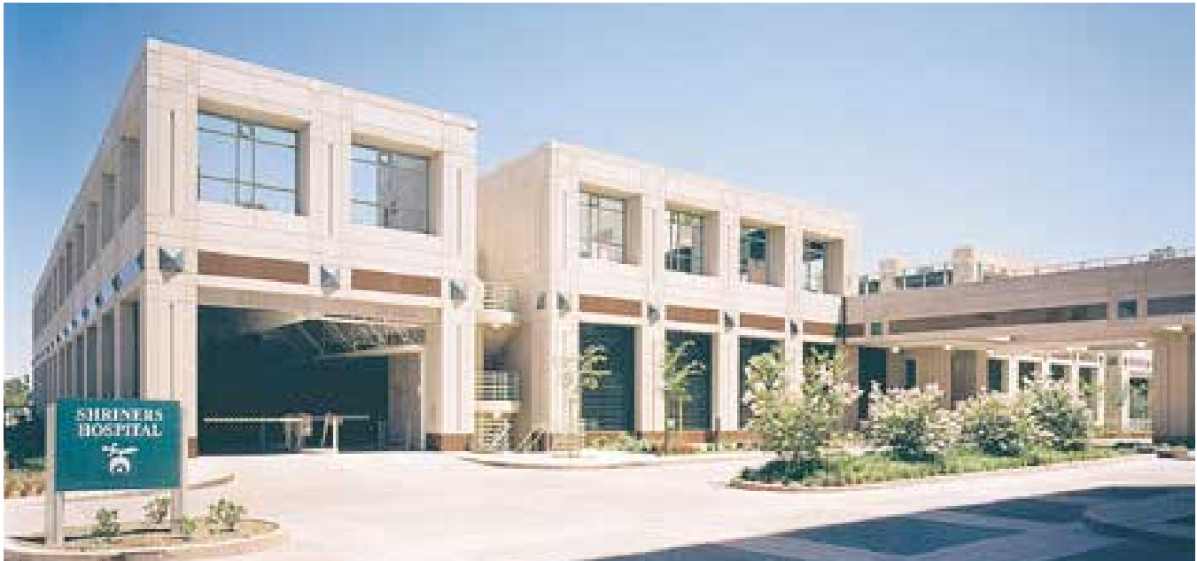
Fig. 2. Adjoining parking structure also features architectural precast panels to complement hospital façade.
