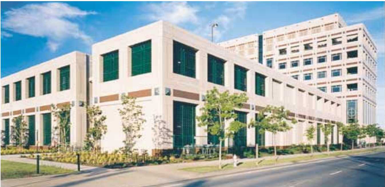
Fig. 15. The adjacent parking structure, which holds 650 cars, features a similar façade design using precast concrete panels on a reinforced concrete frame. The façade for the first two floors of the structure was treated as one unit, creating two-story-tall “bays” in order to reflect the two-story height of the hospital’s entry lobby.
