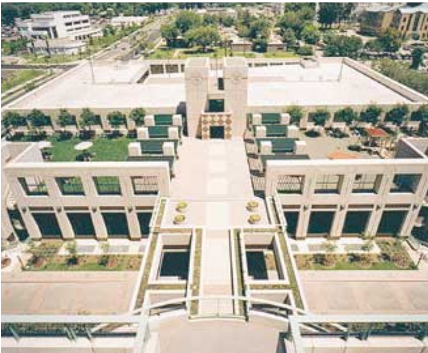
Fig. 16. The parking structure connects to the hospital at its second level via a pedestrian walkway. It was designed as a free-standing structure to aid its seismic resistance.
