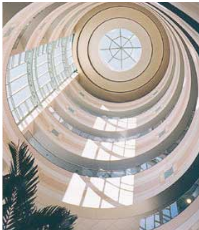
Fig. 13. The atrium inside the entry lobby features gypsum-board walls that were painted to resemble the precast concrete façade panels, including the granite insets and green terra cotta medallions.
