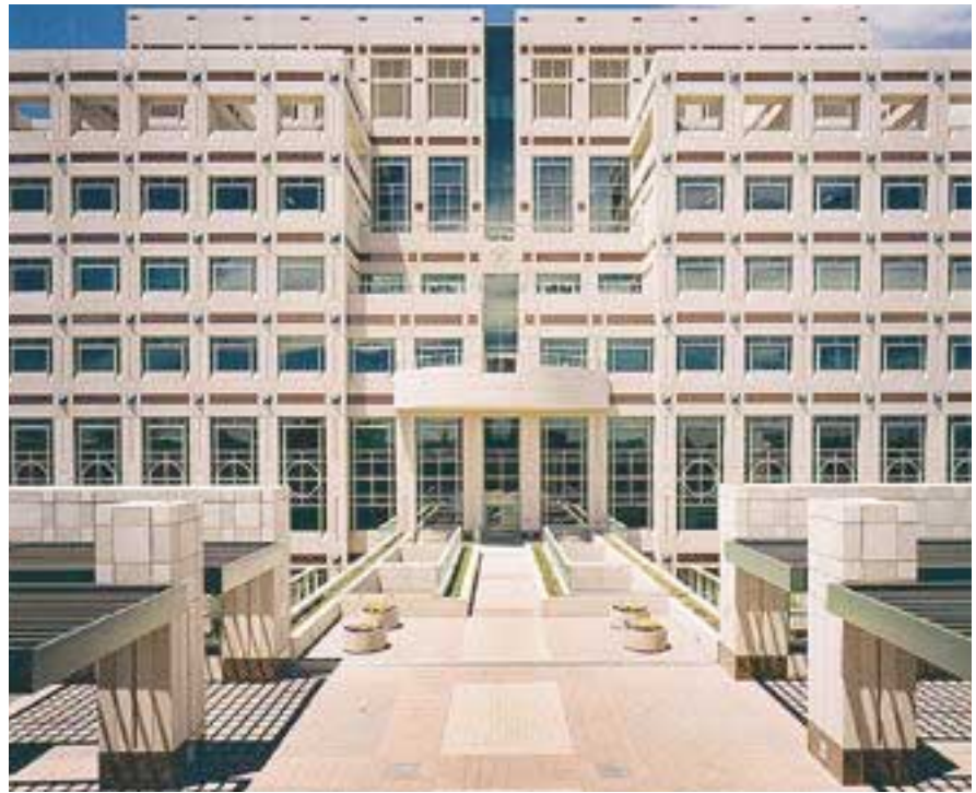
Fig. 6. View from parking structure shows the attractive use of reveals flanking the granite bands and terra cotta medallions.
