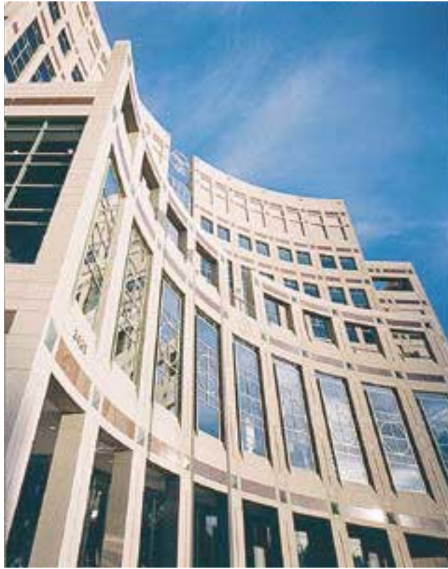
Fig. 8. The curving front façade features the Shriners' logo inset into the center panel, which reflects the logo used at the very top of the building. This circular shape and the pattern in the reveals is mimicked in the mullions in the windows, extending this design theme.
