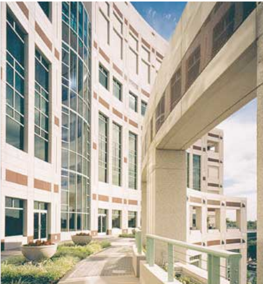
Fig. 12. The arched columns along the lobby's roof combine two panels, one convex and one concave, which are then capped by another precast piece that had to match both inside and outside curves exactly.
