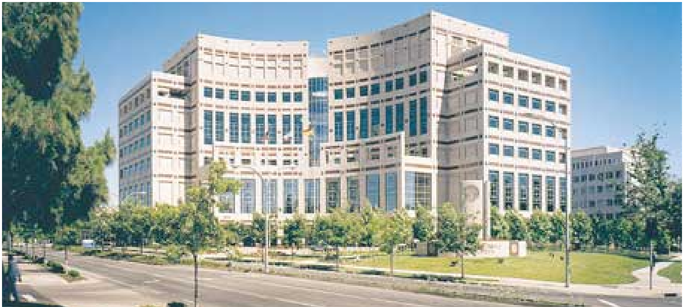
Fig. 1. Shriners Hospital for Children, Sacramento, California. This nine-story building features an exterior façade using architectural precast panels with a horizontal band of red granite, green terra cotta insets and two textures of finish.
