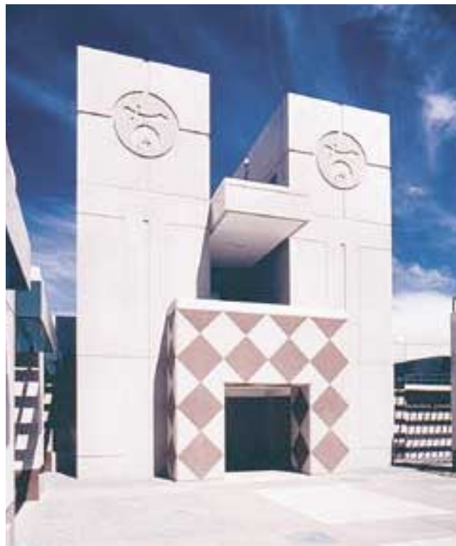
Fig. 17. The elevator entrance panel required casting five individual panels, which then were cast into the main body of the panel. Each casting incorporated a red diamond-shaped pattern to reflect the banding in the hospital.
