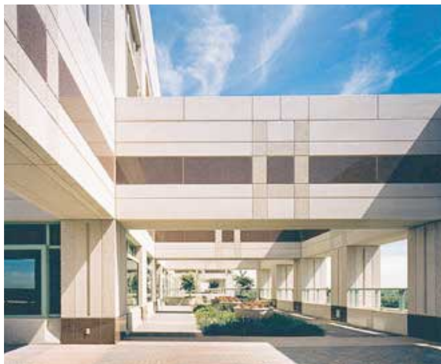
Fig. 14. The variety of textures used in the project can be seen in this view from an upper level balcony. Reveals and two textures of sandblasted finish add visual interest and contrast to the polished granite insets.
