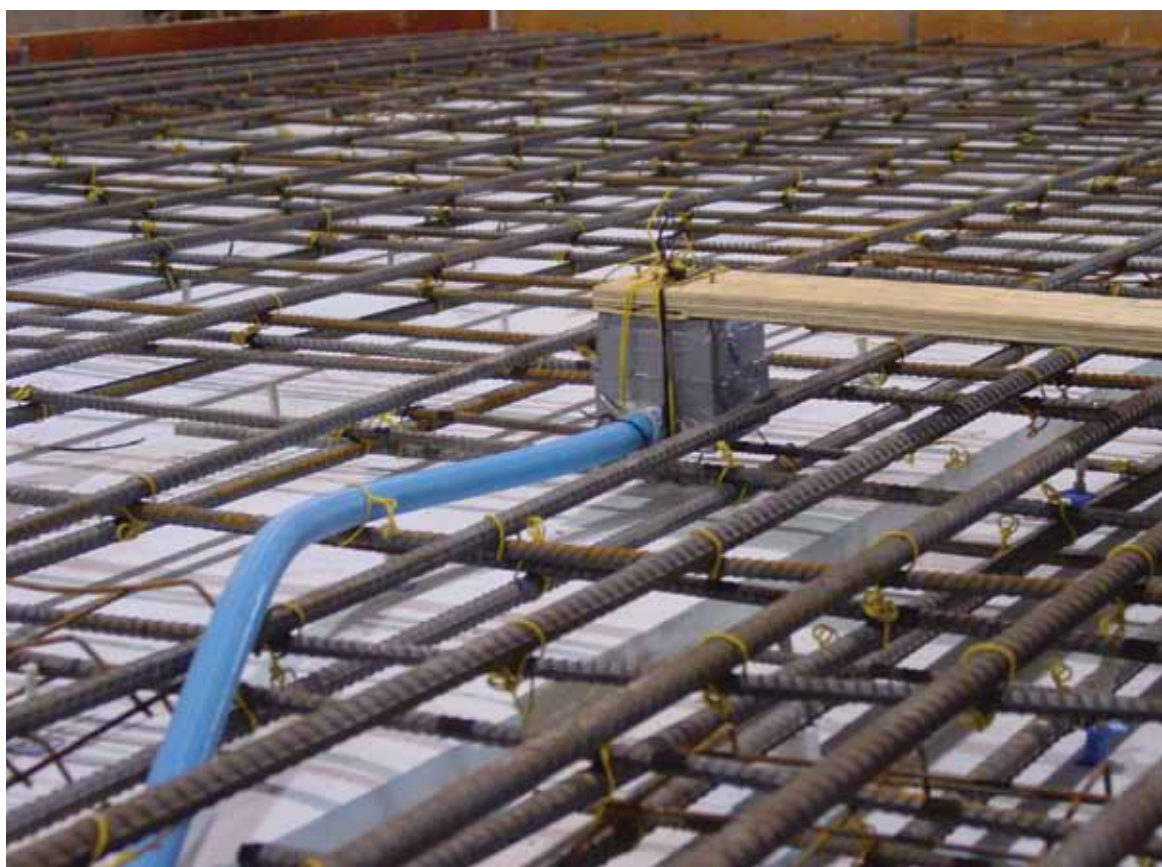
Figure 4 Electrical conduit and outlet box being installed in insulated sandwich wall panel.
