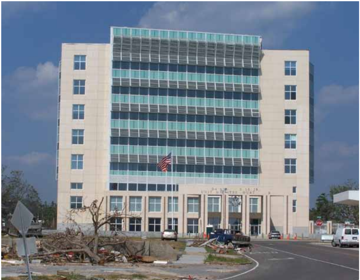
Figure 5 Insulated sandwich wall panels provided excellent protection from hurricane force winds and flying debris.
