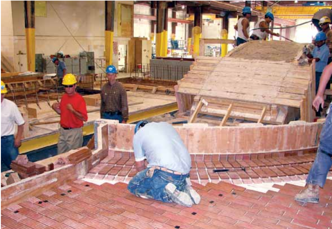
Figure 19 Placing units in form liner (Photo: Gate Precast Company.)
