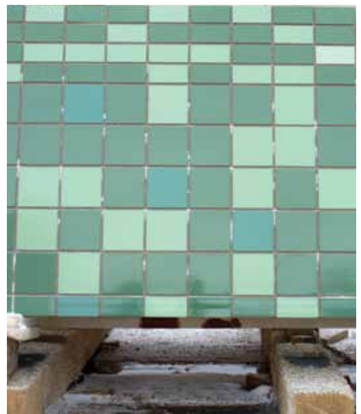
Figure 13 Mercy West Hospital, Green Township, Ohio; Architect: Ellerbe Becket (an AECOM Company), Minneapolis, Minnesota; (Photo: Randy Wilson).
