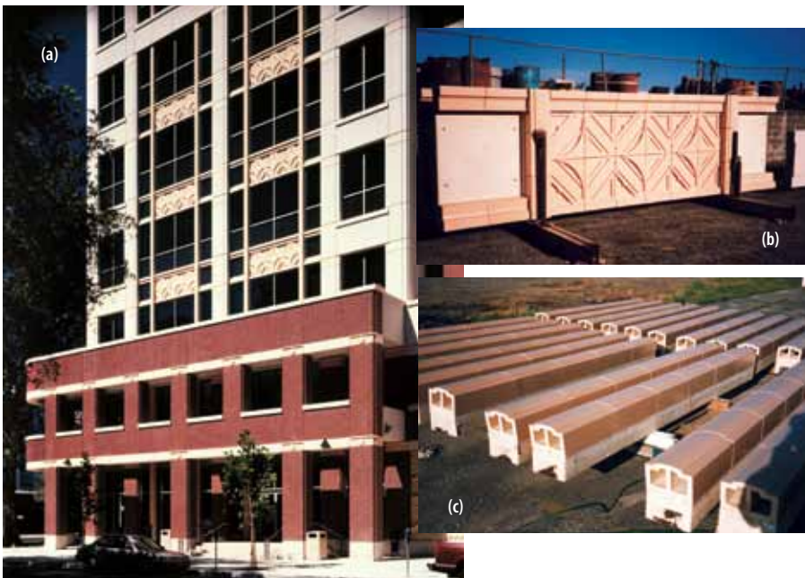
Figure 15 (a), (b) & (c) Sacramento County Systems and Data Processing, Sacramento, California; Architect: HDR Architecture Inc. formerly Ehrlich-Rominger; (Photos: HDR Architecture Inc.)
