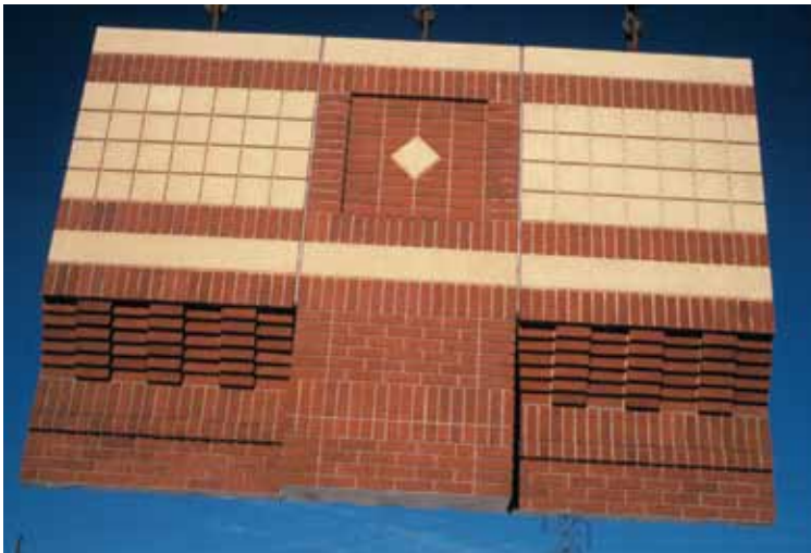
Figure 1 Bonding patterns incorporated into the finished panel.
