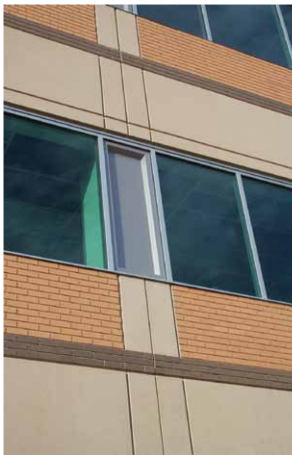
Close-up of orphaned light-colored, thin-brick units at accent field to vertical exposed.
