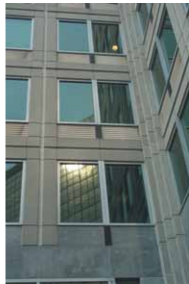
This closeup shows stone clad precast inset accents on high rise office building. Although the building was completed in 1991 the stone has not shown visual evidence of damage due to weathering.
