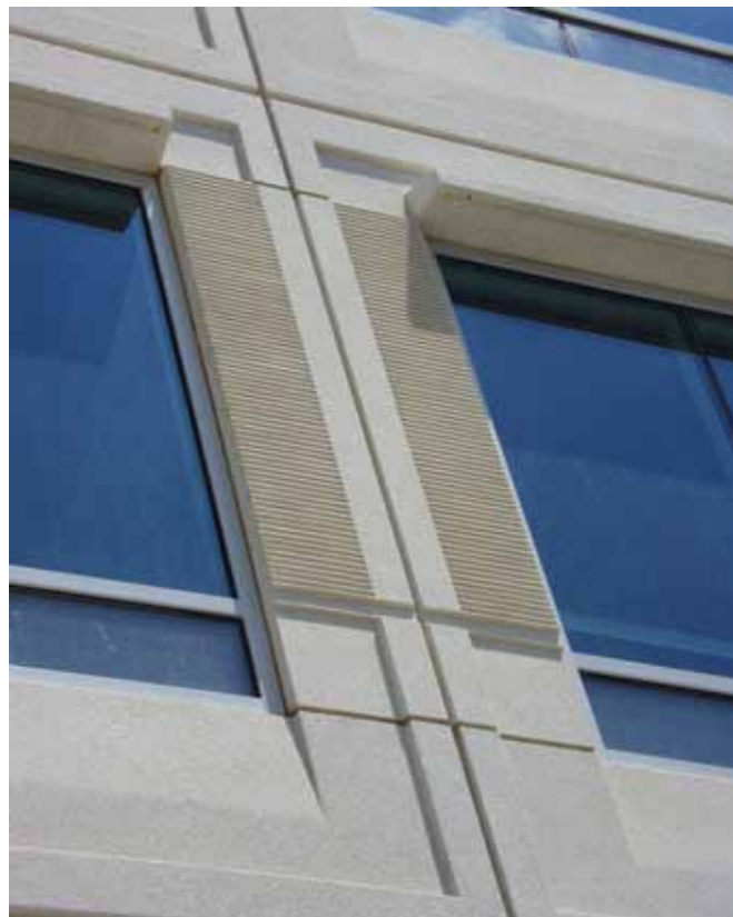
The deft use of modularity, textures, planes, reveals and a single mix design combined with precision craftsmanship in fabrication and erection can render cost effective three dimensional architecture in precast concrete as illustrated in this close-up image at Gensler's Discovery Square Project located in Reston, Virginia. (Courtesy Timothy Taylor)
