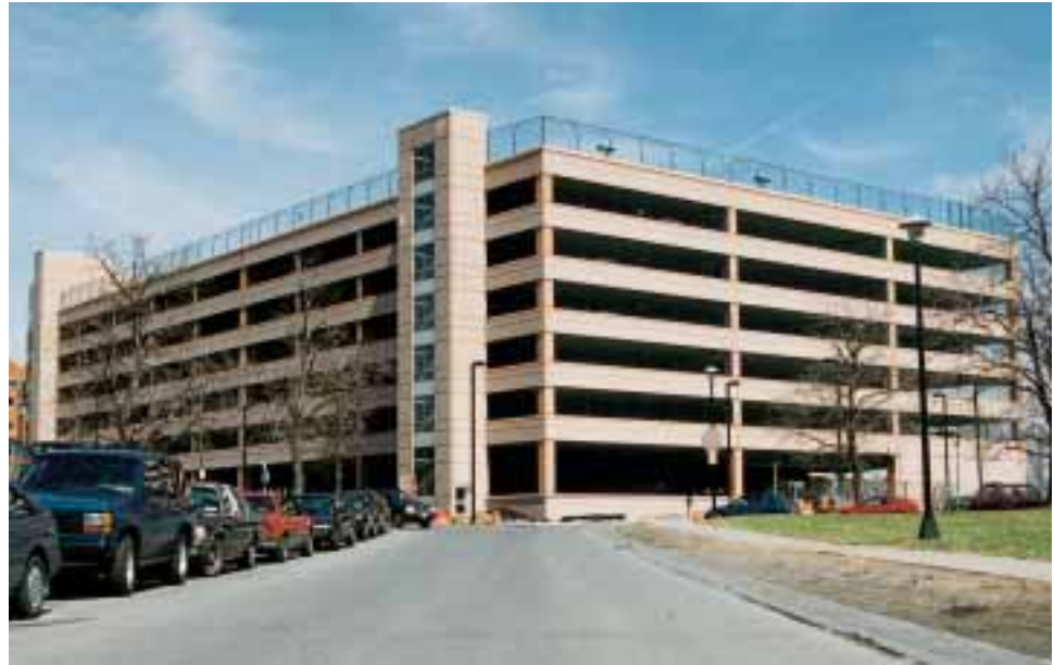
Albany Medical Center Parking Structure, Albany, NY
