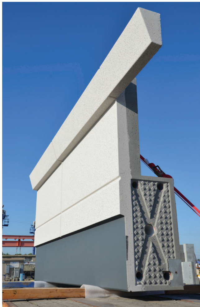
All-in-one where finishes are integrated into structural systems. Enhanced performance and resiliency is provided through the use of the Precast Hybrid Moment Frame.
