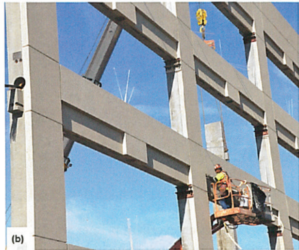
Fig. 6: The Roseville City Hall Annex included integrated architectural finishes on a PHMF structure: (a) view of the completed building ( photo courtesy of John Swain Photography ); and (b) a view of the erection of the exterior frame. Post-tensioning strand extensions can be seen at the leftmost column ( photo courtesy of Clark Pacific )
