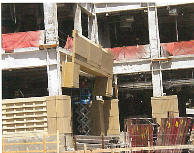
Fig. 1: Typical architectural precast cladding is installed after the building frame has been erected (and, in this case, fire-proofed). “Archi-structural” precast framing eliminates these activities from the construction schedule (photo courtesy of Clark Pacific)
