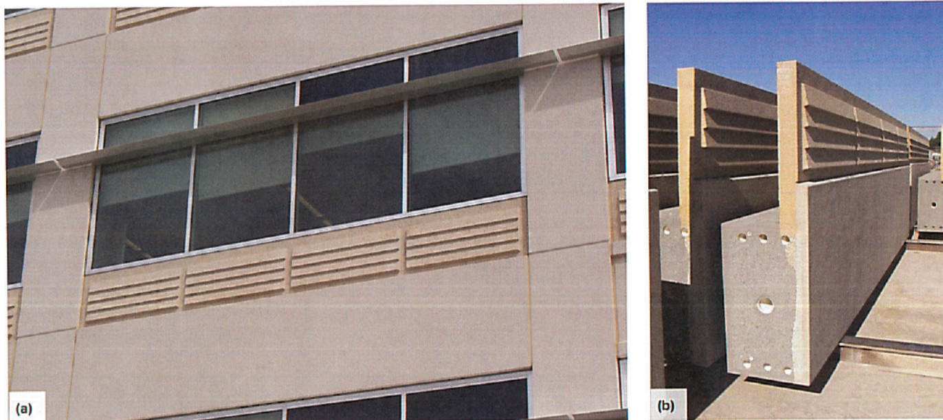
Fig. 5: Precast elements for the Caltrans District 3 Headquarters façade were fabricated with multiple finishes: (a) the PHMF structure provides wide-open window areas with no bracing or solid panels; and (b) an end view of a spandrel panel shows how different concrete mixtures were layered to create a structural element with two distinct architectural finishes (photos courtesy of Clark Pacific)
