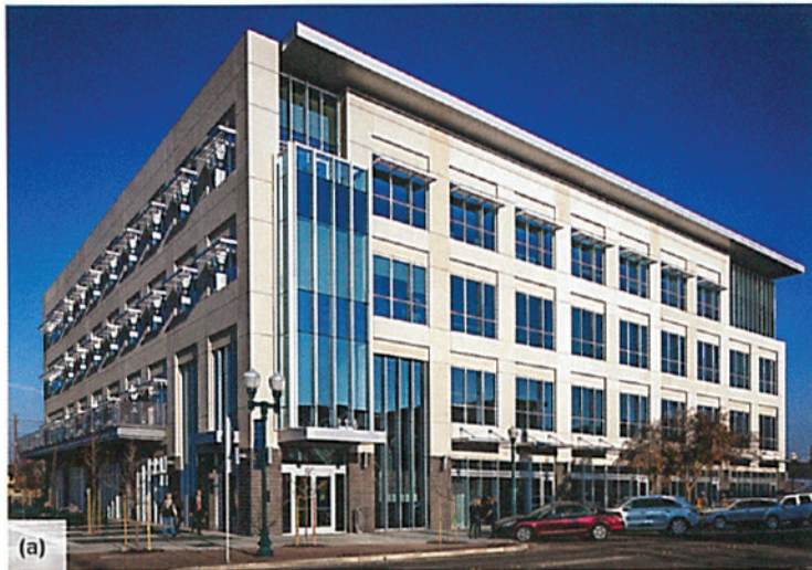
Fig. 6: The Roseville City Hall Annex included integrated architectural finishes on a PHMF structure: (a) view of the completed building ( photo courtesy of John Swain Photography ); and (b) a view of the erection of the exterior frame. Post-tensioning strand extensions can be seen at the leftmost column ( photo courtesy of Clark Pacific )
