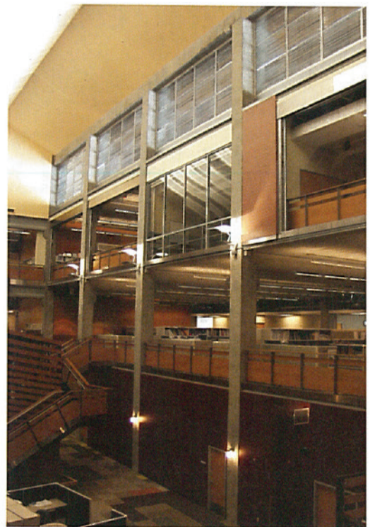
Fig. 4: Incorporating PHMF into the Caltrans District 3 Headquarters design allowed the designers to deliver a wide open and well-lit interior (photo courtesy of Clark Pacific)
