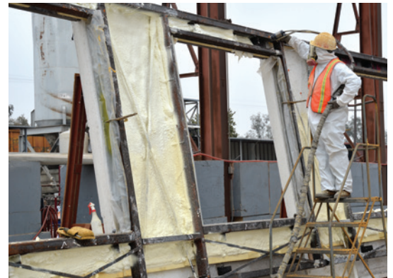
Applying spray foam insulation to the panel
