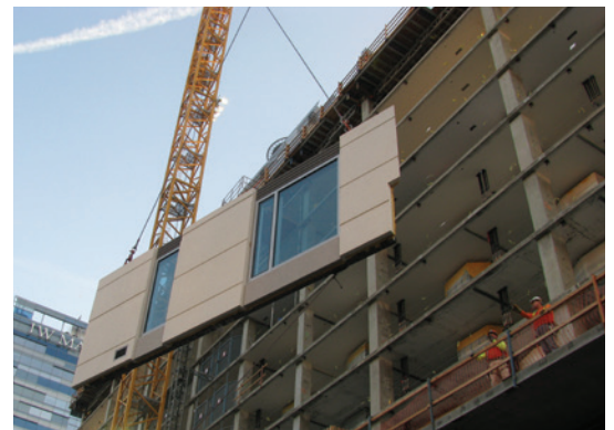
Complete prefabricated units installed at jobsite
