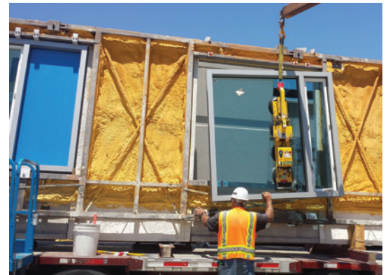
Installing glass in a pre-insulated panel
