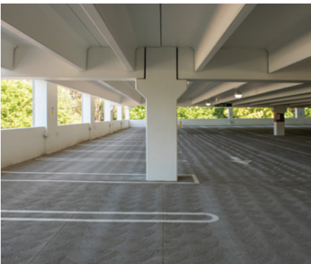
Use of the Precast Hybrid Moment Frame gave the structure an open plan for safety.
