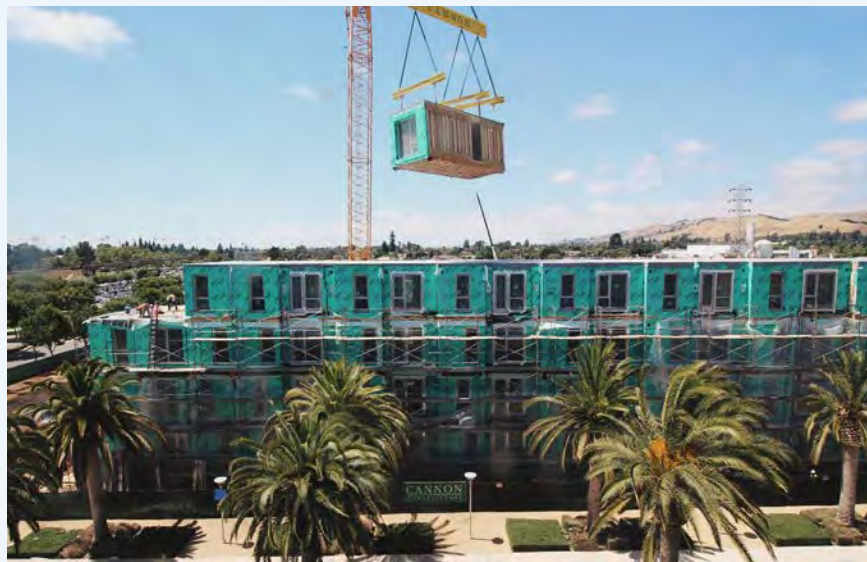
The Union Flats features 388 wood-framed modules, craned into place at a rate of 12 per day.
