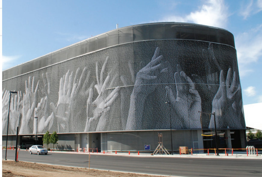
The structure's east façade features dramatic full-length murals that were decided on after the precast had been erected. Embeds in the spandrels allows the artwork to be attached after construction.
