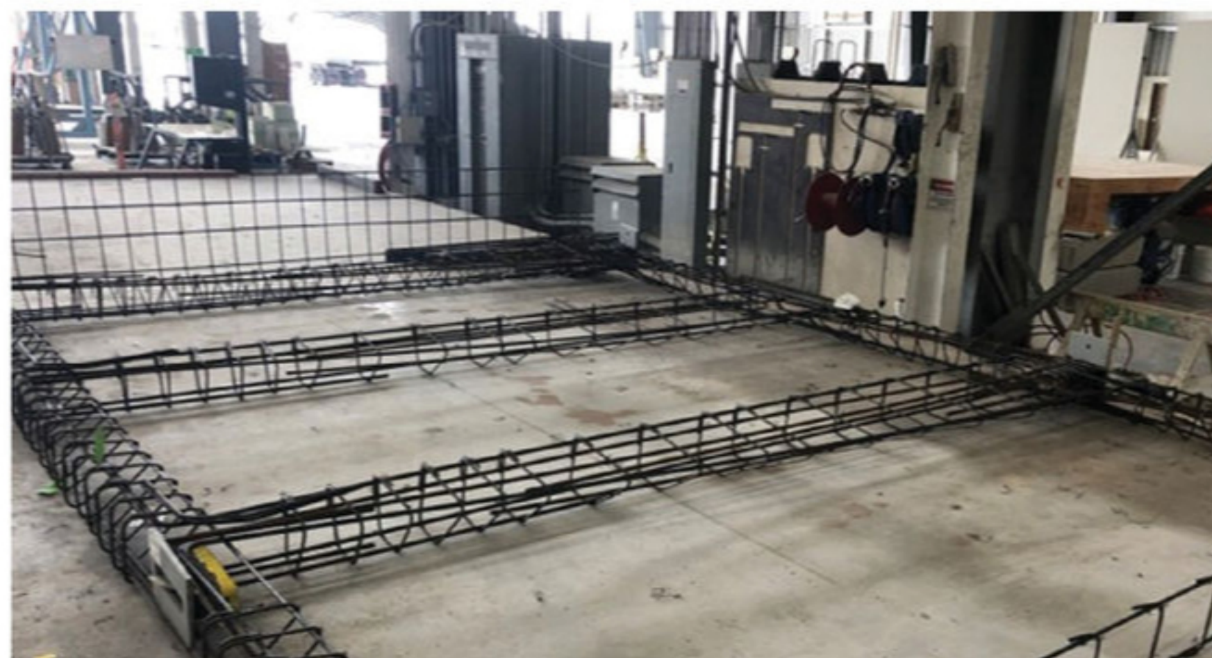
Mission Rock G rebar cages at Clark Pacific’s yard, ready for production.
