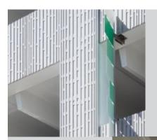
Utilizing form liners, the facade of the structure was designed to mimic tree bark to blend with neighboring arboretum.
